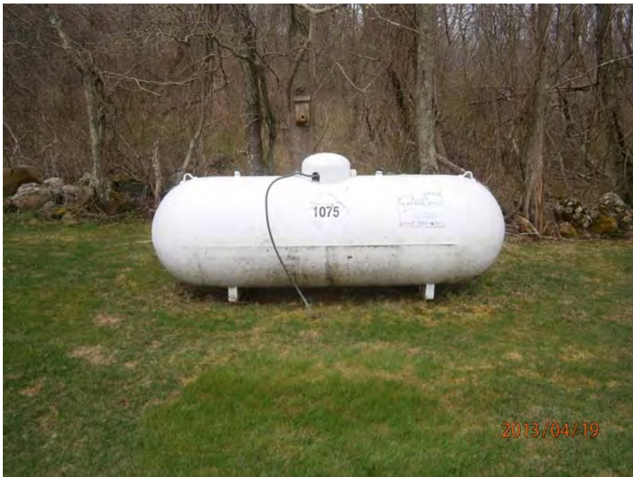
19. Generator fuel storage tank
